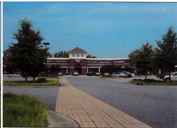
Main pedestrian access in Oak Ridge Commons
