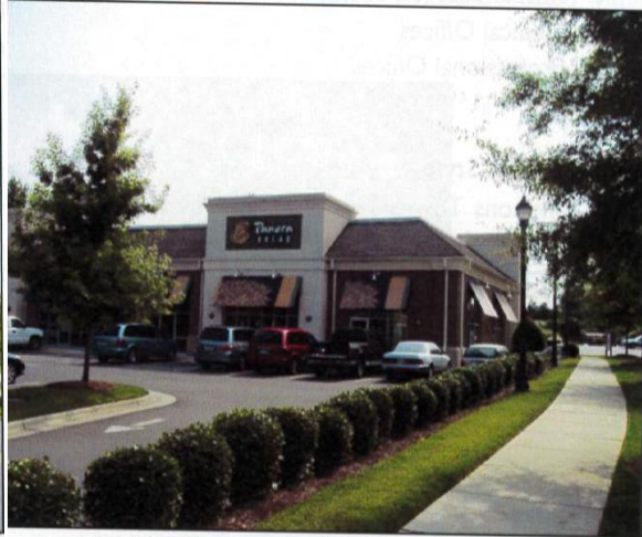
Brick façade, pitched roof, and stucco entrance way
